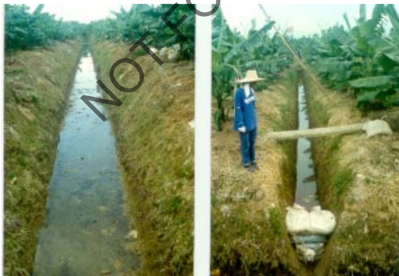
Fig. 5. A minidam (left) to impound water in a drainage canal, and an adequate supply of impounded water (right) during El Niño.
